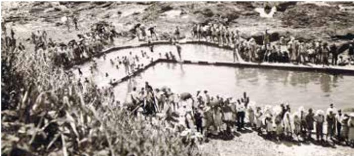
This iconic pool was first constructed in 1940. It is 100 feet long and 30 feet wide (30m x 9m) and was built by local bridge and road contractor, Mr M Milligan, at a cost of £500. It was re-concreted in 1945.
